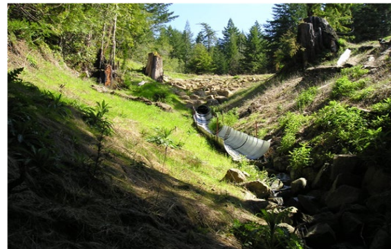
Stormproofed Stream Crossing – Elk River Watershed
