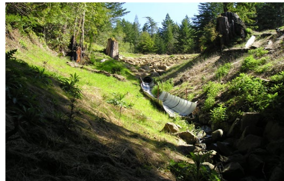
Stormproofed Stream Crossing – Elk River Watershed
