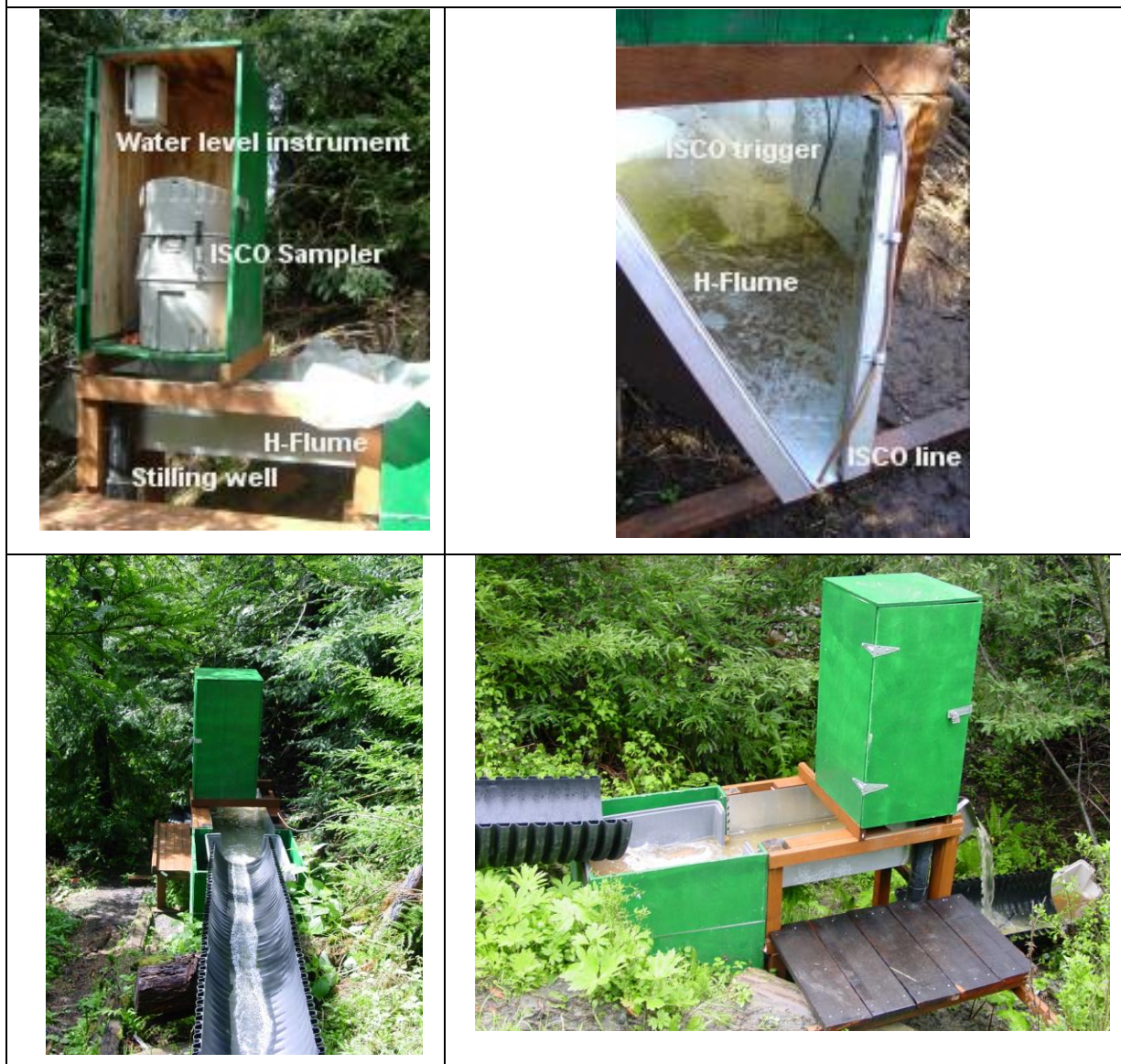
Figure 6. Photos of the flume installations.
