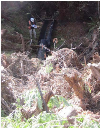
Figure 6. Culvert downspout specification inspection
