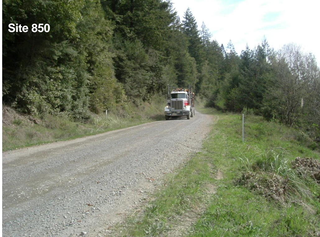
Figure 3. Photographs of road sites on the N. Fork Elk River (ER) mainline road, measured in 2004 and 2005. Site 850 was 7.5% gradient and 851 was 17% gradient.
