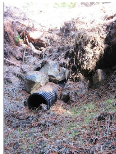
Figure 19. LWD chunks keyed into culvert outlet fillslope.
