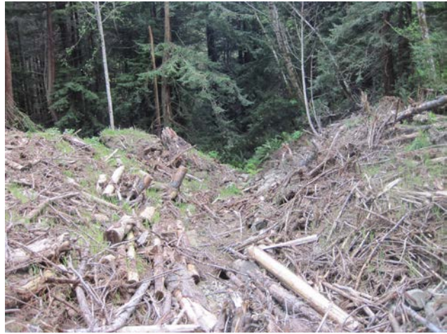
Figure 25. LWD placed in pulled stream channel.
