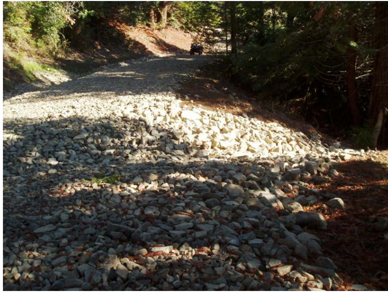
Figure 12. Newly constructed Class III rocked ford.
