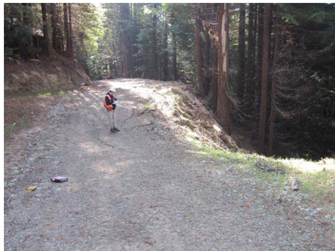
Figure 3. Wet weather Inspection of culvert crossing
