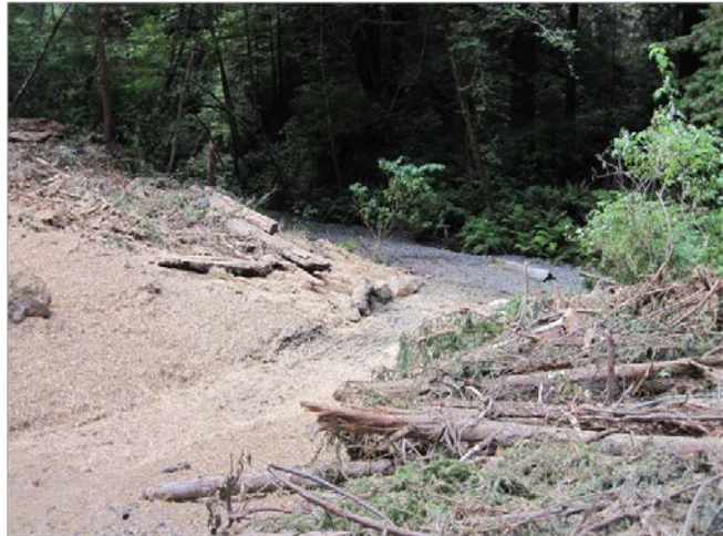
Figure 2. Newly excavated closed crossing adjacent to Graham Gulch, Freshwater Creek.
