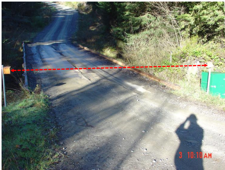
Figure 9. Photograph of traffic counter installation.
