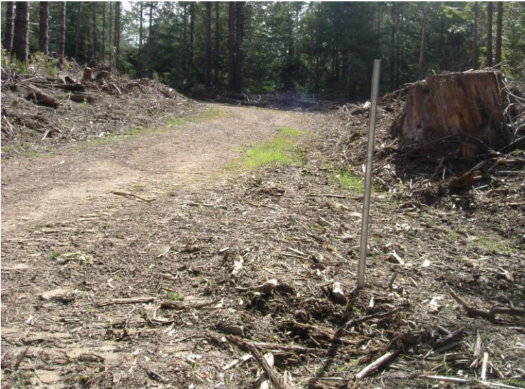
Site 854 Secondary native surface road U91.24 Gradient 15.0%
