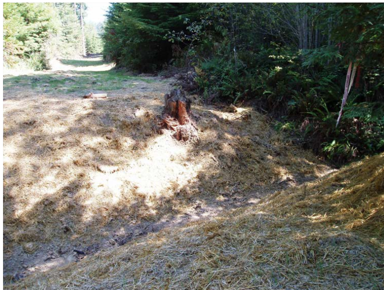
Figure 21. Newly pulled Class III closed crossing
