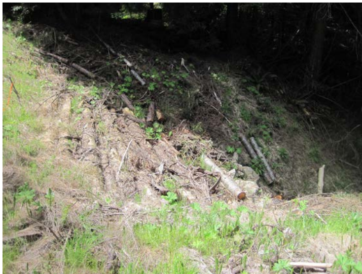
Figure 18. LWD cribbing along outlet fillslope of culvert crossing.
